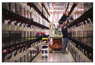
the delivery of electricity from power plants in Anchorage, about 350 miles away. Although the GVEA battery system was initially configured with four strings, it can readily be expanded to six strings to provide a full 40 MW for 15 minutes. The facility can ultimately accommodate up to eight battery strings, giving flexibility to boost output or prolong the useful life of the system beyond the planned operation for 20 years.
