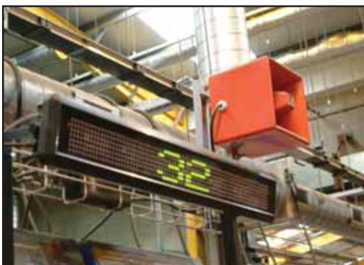
iBOS Display and Shouter: The iBOS Display eliminates truck operator confusion by identifying which battery should be taken next. The Shouter sounds an alert when an incorrect battery has been taken.
