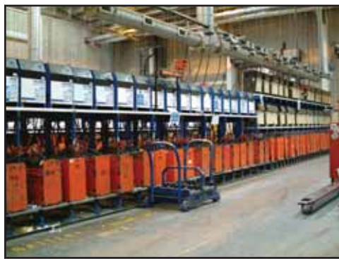
Wakefield Battery Room: Chargers (top) and batteries (bottom); a manual battery changer is used to exchange batteries.
